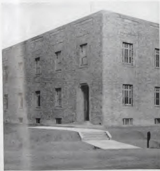
American Telephone and Telegraph Co. Repeater station, Ridgeville, Ohio Mills, Rhines, Bellman & Nordjoff, Architects, Toledo, Ohio W. J. Schirmer Co., Contractors, Cleveland, Ohio Medusa Waterproofed Gray Portland Cement used in all floors, foundations and for brick mortar.
